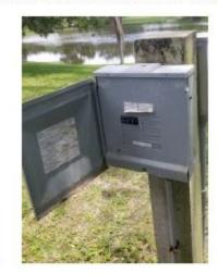
c. Move Sprinkler Controller from back of sign to concrete post that houses circuit breaker
