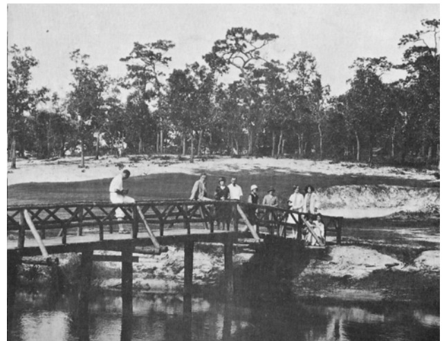
Dunedin Golf Course bridge at 11 th hole
