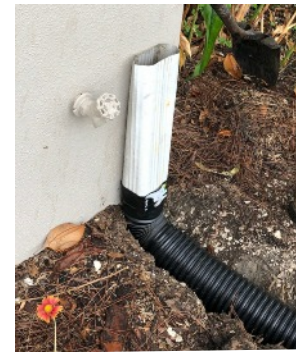
Pipe attached to downspout
